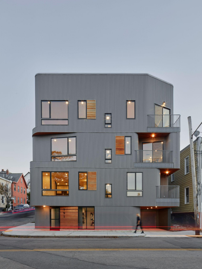
Condor Housing - Flats East Boston, MA 9-Unit Multifamily Housing
